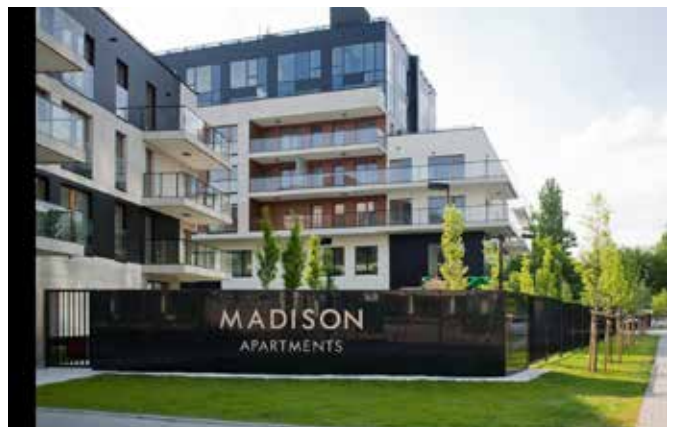
Madison Apartments - Poland - Clima Canal
