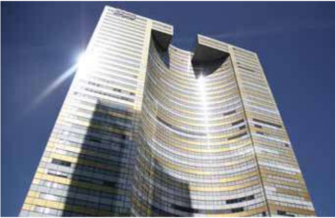
Tour Eqho - France - Clima Canal
